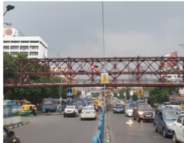
Dhakuria Foot-over bridge during retrofitting, Kolkata, India, Progressive Construction
