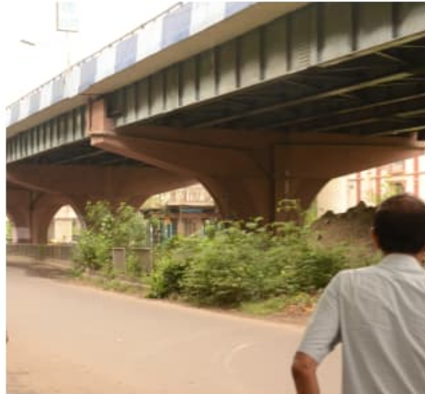
Wipro Flyover Inspection, Kolkata, India
