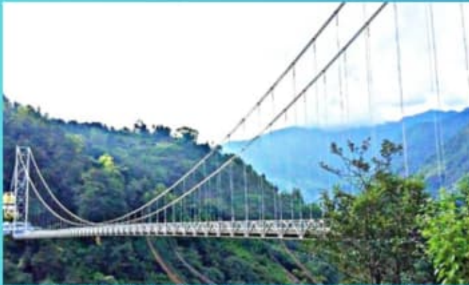
Singshore Bridge Restoration, Sikkim, India, PWD
