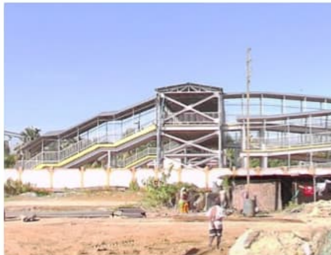
Jagiroad Station Foot-over bridge, Assam, India, NF Railway
