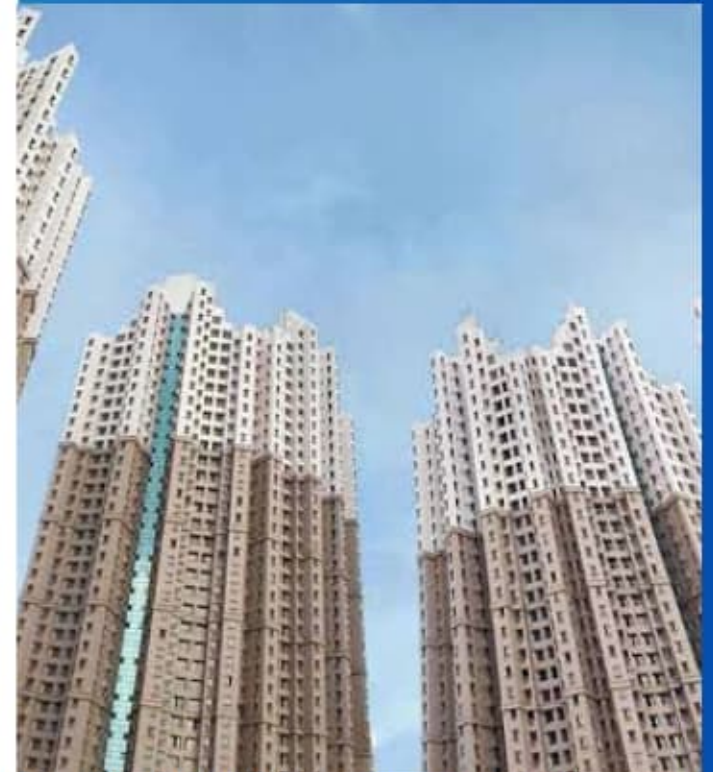
South city buildings assessment, Kolkata, India
