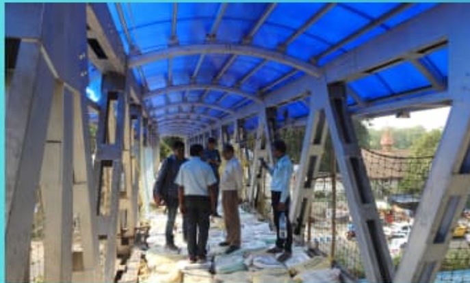
Monitoring Load testing of Alipore Foot-over bridge, Kolkata, India, Kolkata Municipal Corporation
