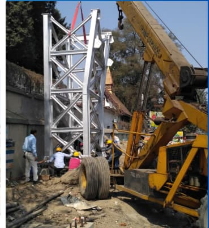
Trestle Erection inspection of Alipore FOB, Kolkata, India, Kolkata Municipal Corporation
