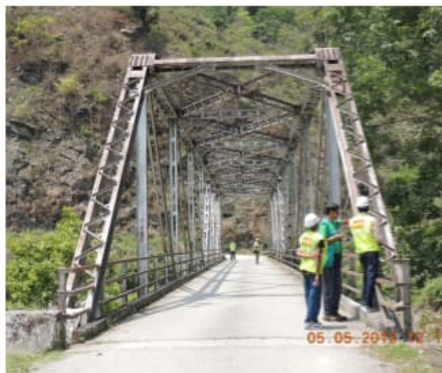
Inspection and assessment of Bridges, Sikkim, India, PWD
