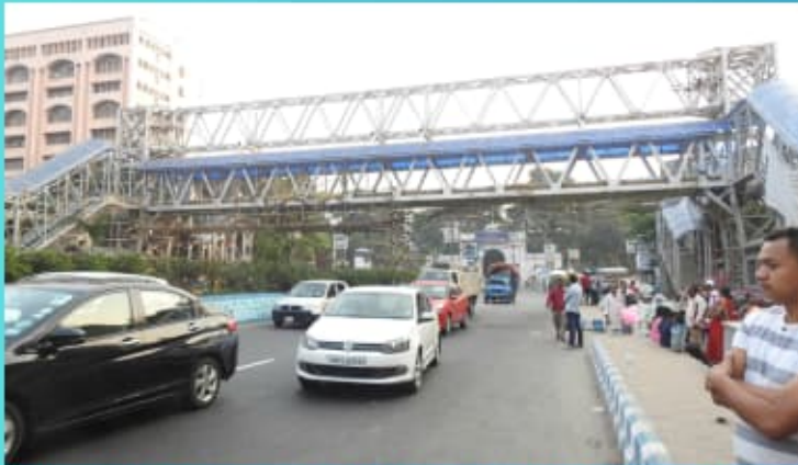
Alipore Foot-over bridge, Kolkata, India, Kolkata Municipal Corporation
