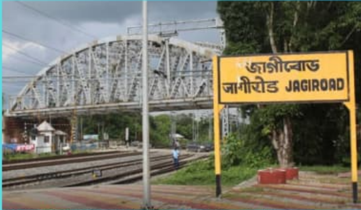
74m Rail over bridge, Jagiroad, Assam, India, NF Railway
