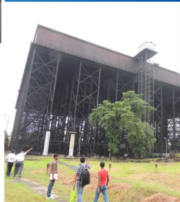
Tallah Tank, Retrofitting & Rehabilitation, Kolkata, India, Kolkata Municipal Corporation
