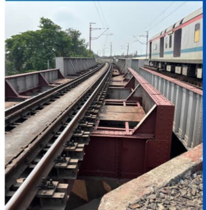
Re-girding of Railway bridges, Kolkata, India, Eastern Railway
